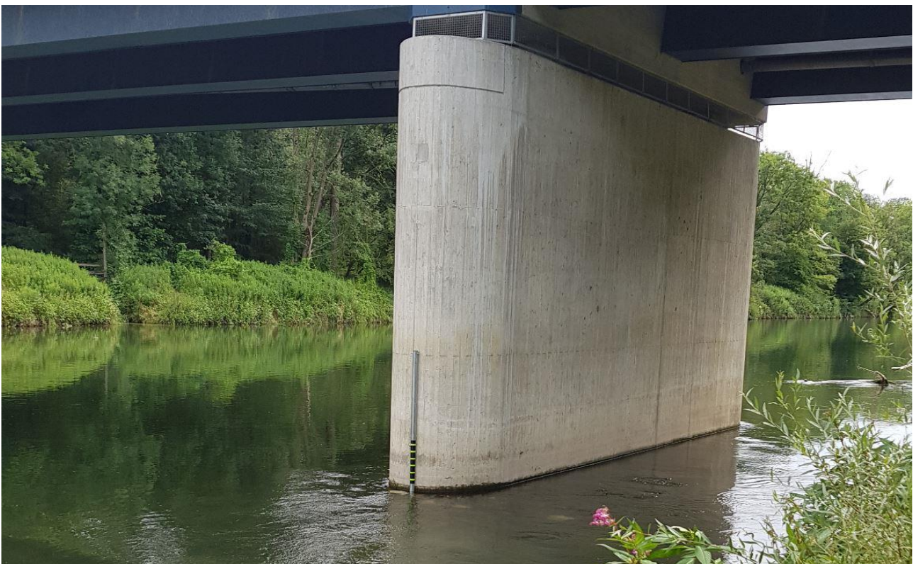
Figure 4: The newly installed gauging station in the Isar river in Neufahrn bei Freising.
