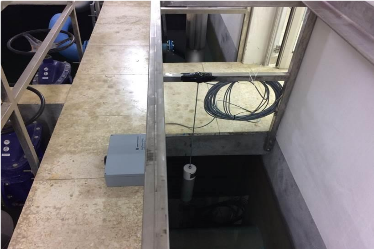
Figure 2: Installed multi-parametric probe in the Neufahrn bei Freising pilot area.
